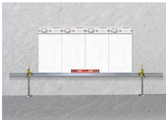
Aluminum bar supports the tiles during paneling process
